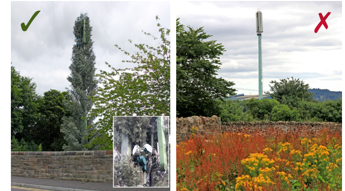
Good example of disguised equipment
