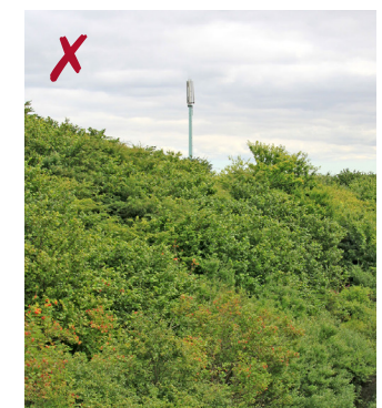
Bad example of monopole location
